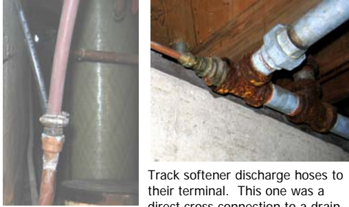
Hose to tube, up to connect to drain.
